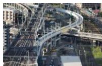
A new inbound approach track at Fukushima Station
