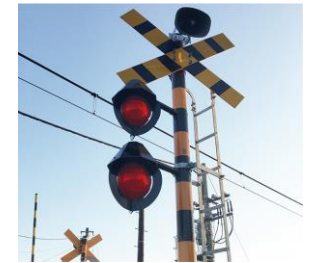
Installing omnidirectional warning lights
