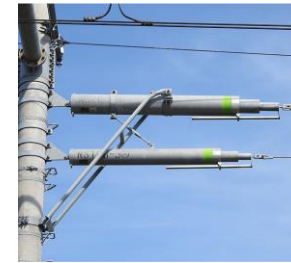
Upgrading overhead wire facilities
