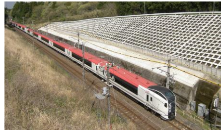
Reinforcing wayside embankments
