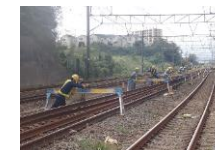
Maintenance and construction during daytime hours
