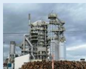
Hachinohe Biomass Power Plant
