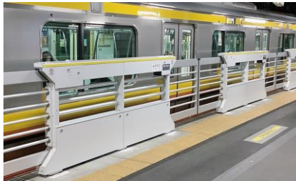
Installing slit-frame automatic platform gates
