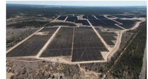
Completed Edenvale Solar Park in Sep. 2023
