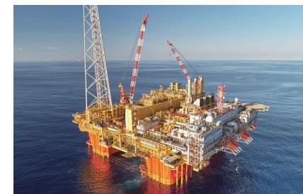
イクシスLNG CPF (Central Processing Facility)
