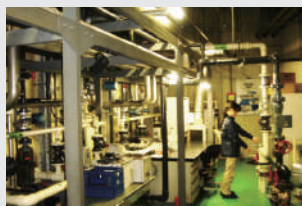
• Greywater plant (kitchen drainage reuse system)
