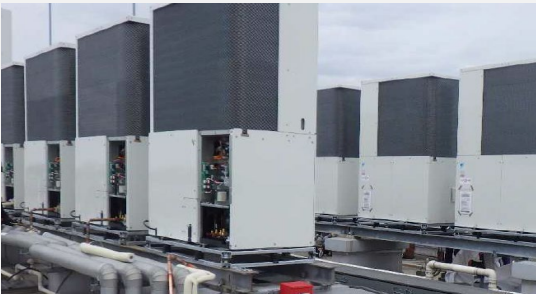
Installation of energy-saving air-conditioning equipment
