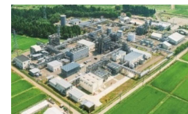
Koshijihara Gas Plant (Niigata, Japan)
