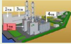
Advancement of replacement of aging facilities of Kawasaki Power Station Unit 1
