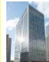
Nakanoshima Central Tower (Osaka City, Osaka)
