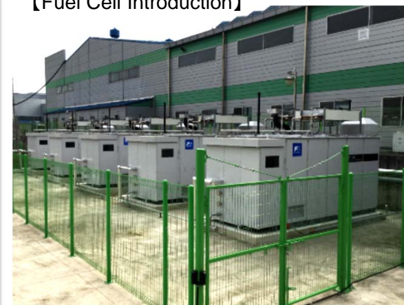
Five 100 kW fuel cells introduced Yuil Industry facility in South Korea (completed in 2017)
