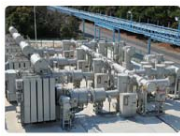
Oil-immersed Transformers
