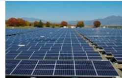
Solar power generation systems
