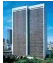
ARK Mori Building
