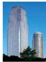
Atago Green Hills (Mori Tower)
