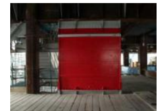
Viscous seismic damping wall
