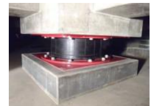
Seismic isolators
