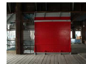
Viscous seismic damping wall
