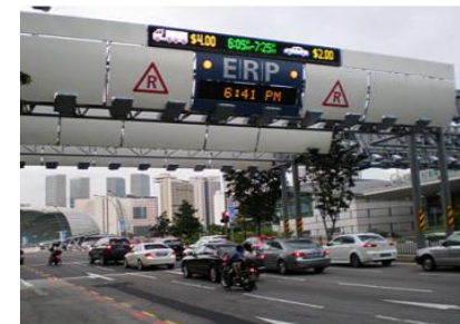
Electronic Road Pricing system(ERP) (Singapore)
