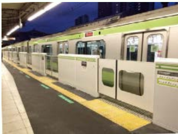
Automatic platform gates installation
