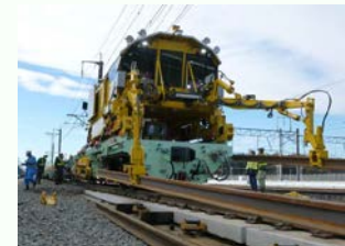
Rail replacement on Tohoku Shinkansen Line
