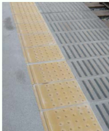
Dot-Braille blocks indicating platform edge
