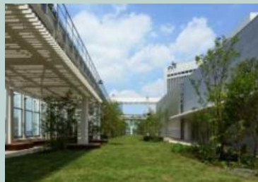
Rooftop garden "sky park"
