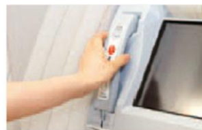
Audio-guidance (from Nov. 2007) Operations possible via intercom, enabling use by disabled people
