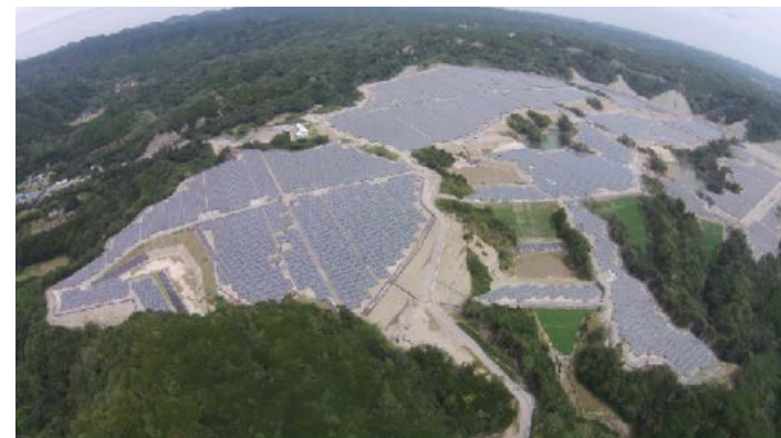
Solar power plant site (Chiba Prefecture)
