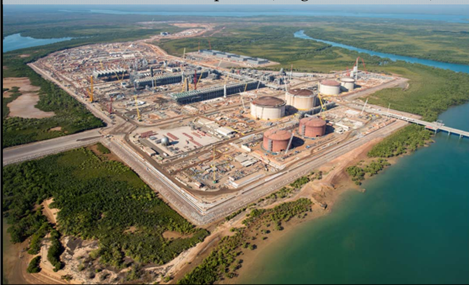
Construction of LNG plant (Aug./2015, Darwin)
