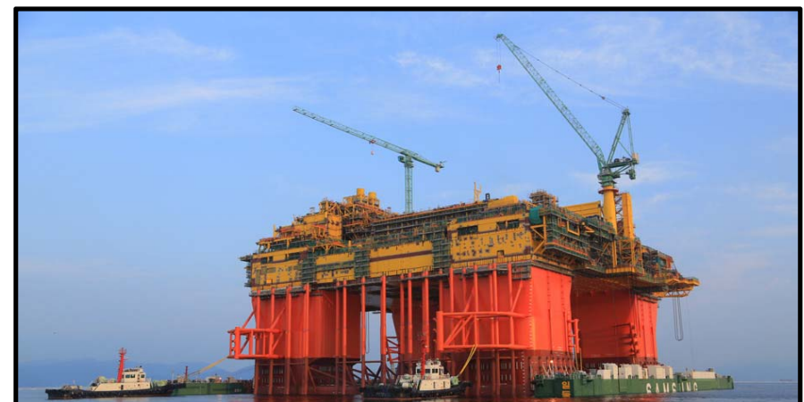
Launched central processing facility (September/2015)
