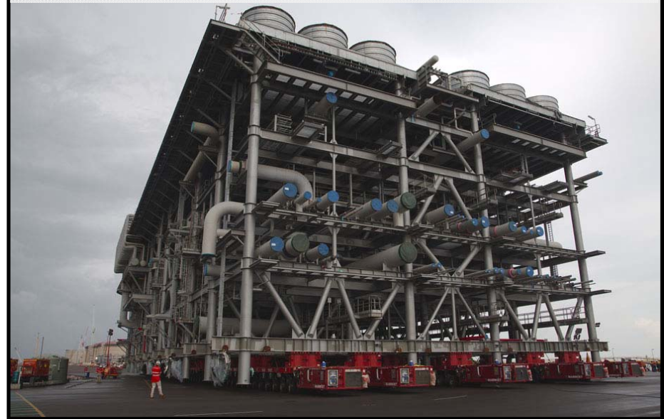
Installation of CPF topside module (April/2015, Korea)
