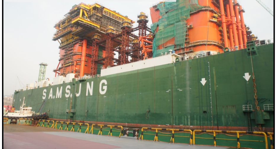
Installation of CPF topside module (April/2015, Korea)
