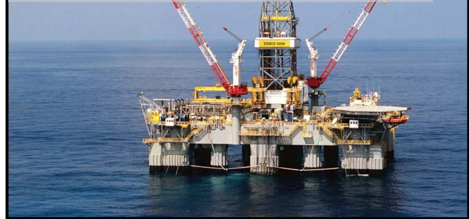
Commencement of drilling of production wells (February/2015)
