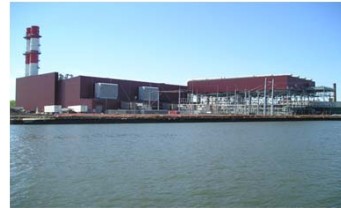
IPP(US: Astoria I gas power plant)
