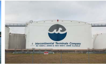
US: tank terminal for chemical products
