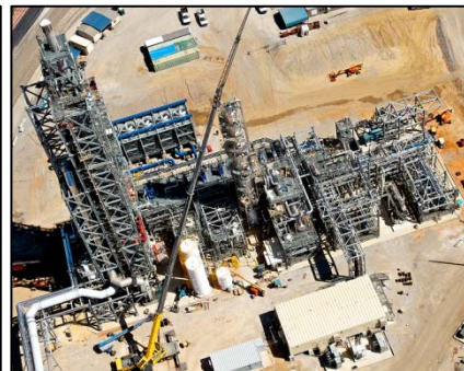
2011: 500 ton/day United States <CCS demonstration at coal-fired power plant>
