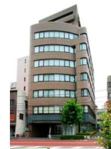
Ueno Takeuchi Building
