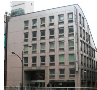
Rosebay Shinjuku Building
