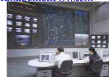
Traffic/Road Management System
